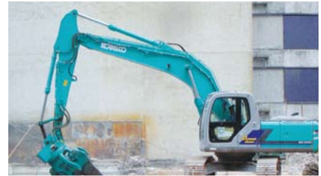
Hydraulic crushers reduce noise during construction.
